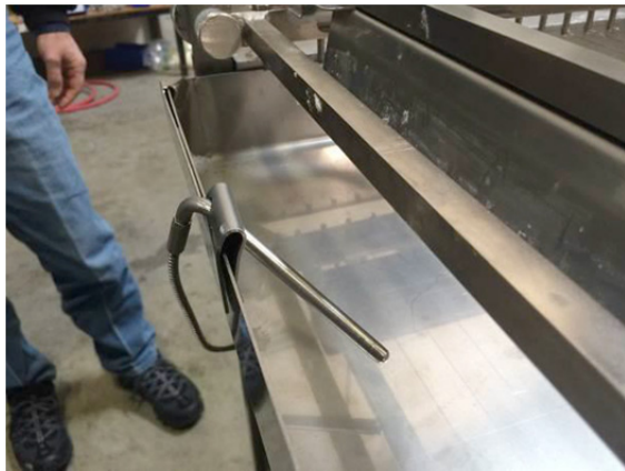
Figure 7, Installation of Thermocouple
